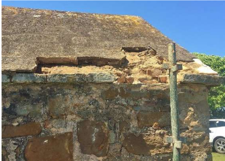
Left: Repairs to roof (Photo: Tom Barrett)
