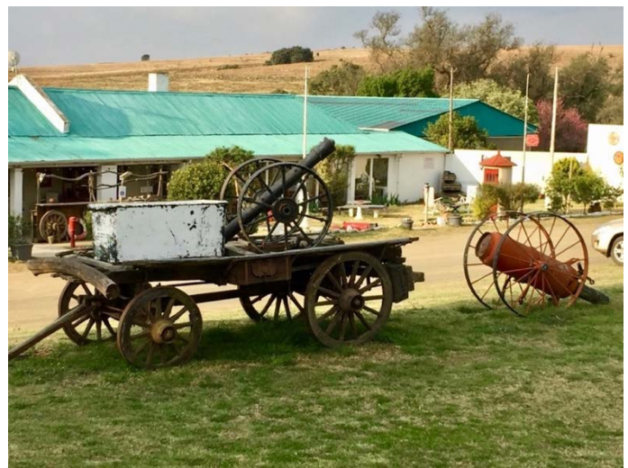
Above: The sea-green roofed hotel (Building 4) with old fire-fighting equipment in the foreground (Photo: Sue Gordon)
